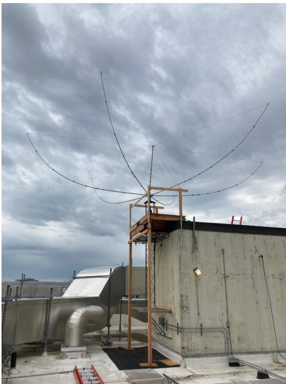
Figure 10: MFJ-1848 antenna on the roof of Buckman Hall
